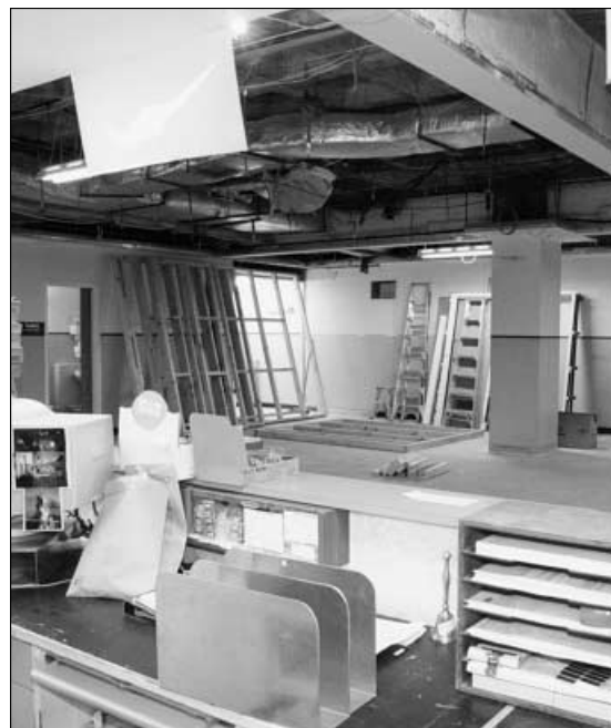
A reception area under construction.
